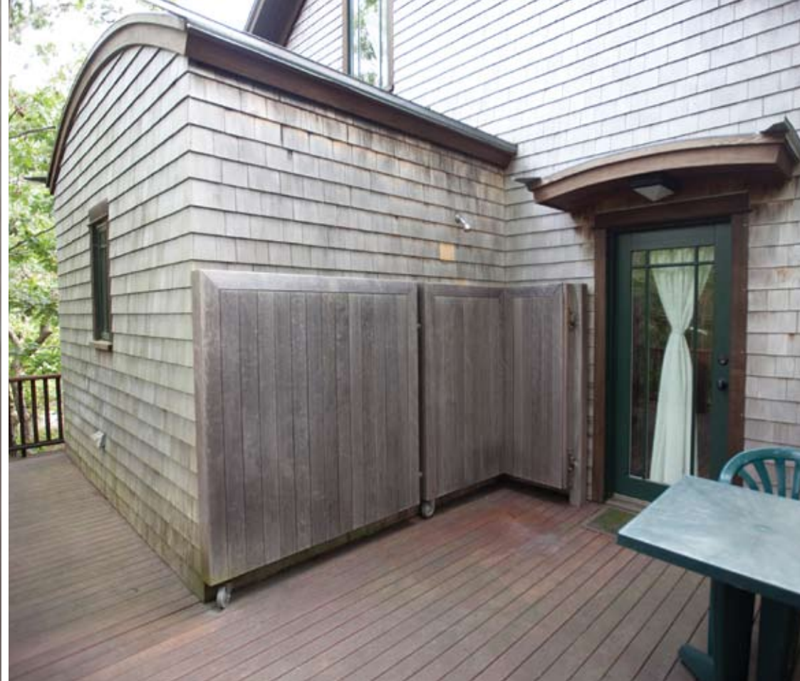
Ben Kelley designed this “disappearing shower” in Oak Bluffs to save space – the walls roll out from the house when you’re ready to use the shower.
